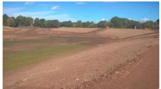
Construction of the embankment
