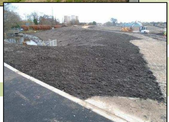
Top soiling of grasscrete on the spillway is complete.
